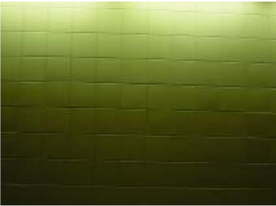
Anyone recognize this? It is a wall at the Tram Platform in McCarran Airport, Las Vegas. It shows the affect of shadowing on a well-installed wall with wall-wash lighting.
